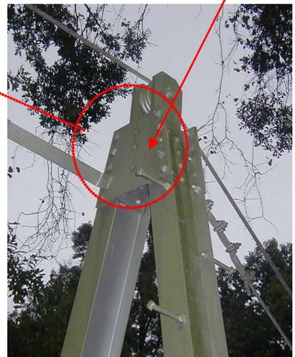
Studs used to facilitate the installation of the Controller & Motor Drive to the Bracket
